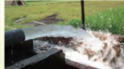
Solar Powered Irrigation System
